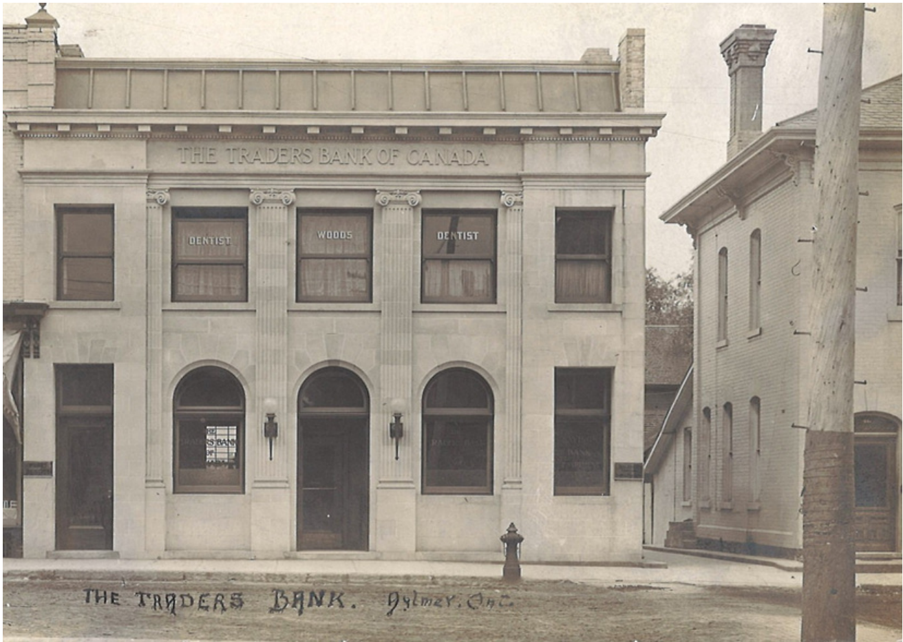
Photograph of the Aylmer Branch of the Traders Bank of Canada, located at 75 Talbot Street East, taken ca. 1909. We are grateful to have the opportunity to house our museum and its ever-growing collection in such a beautiful and historically significant building.
